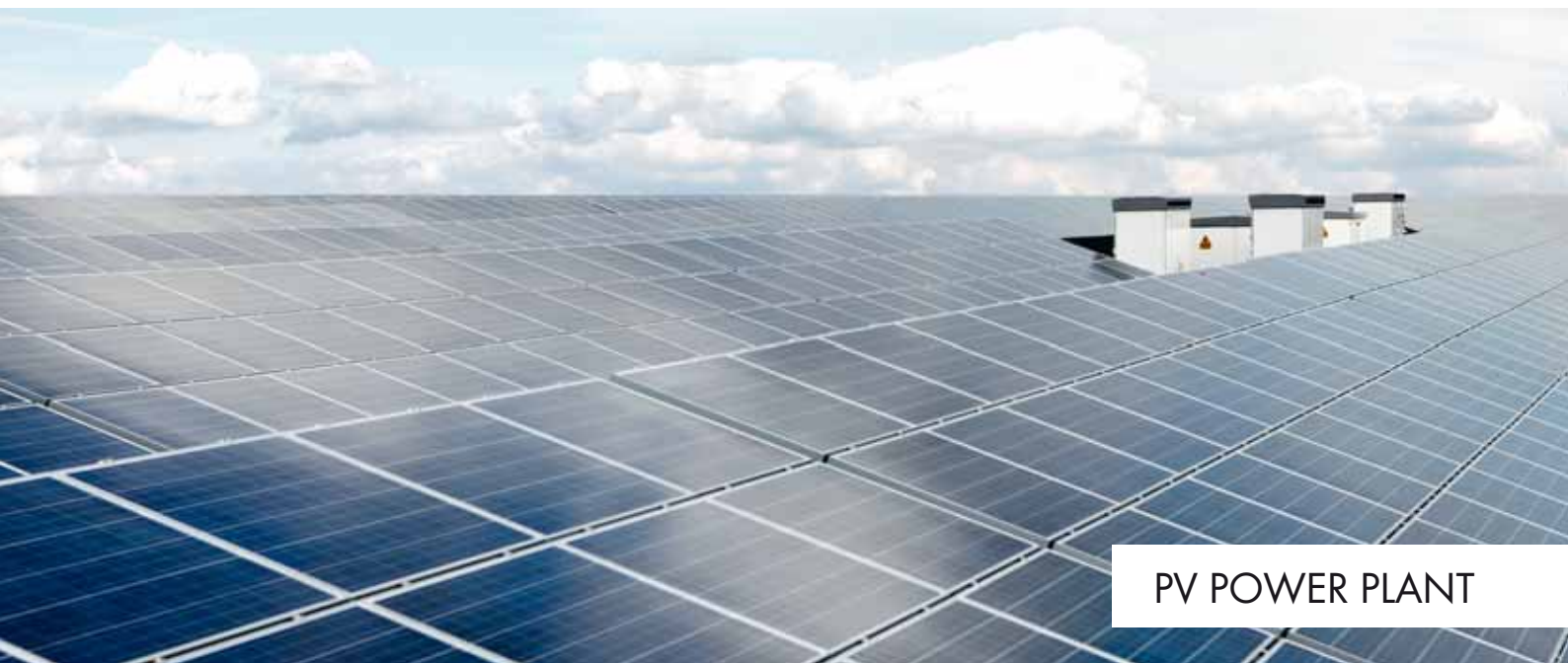
COMMERCIAL PV PLANT
